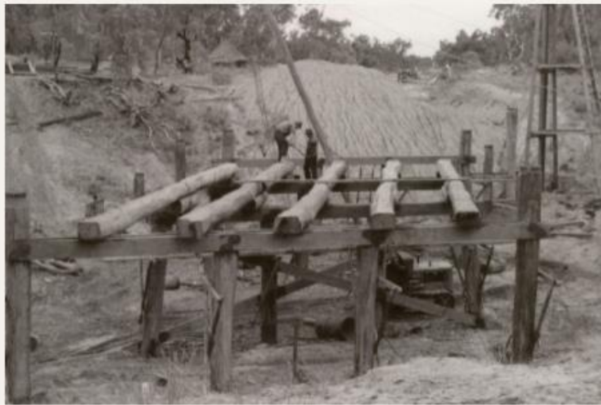
Figure 6.21: Gin pole is at rear centre with ropes extended to place a girder log, with piling derrick at rear (R). Source: Roads and Maritime
