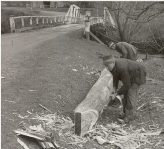
Figure 6.12: Hewing a log with a broad axe. Source: VicRoads, Roads and Maritime copy
