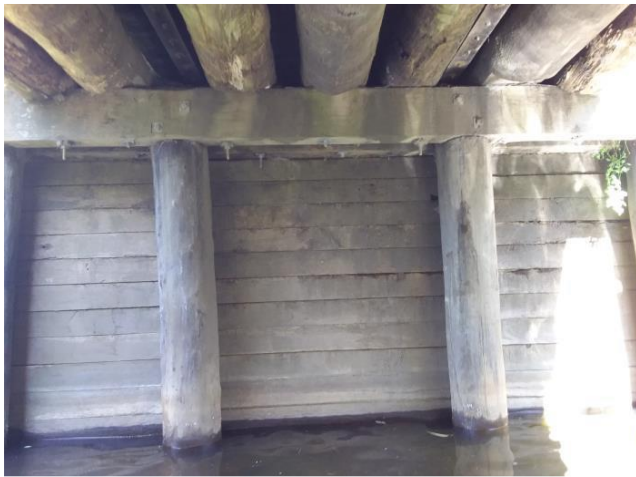
Figure 10. Western abutment. Note redundant girders have been left in-situ (Shoalhaven City Council,, 2021)
