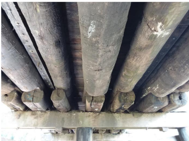
Figure 12. Detail of girders and corbels on the first span (Shoalhaven City Council,, 2021)
