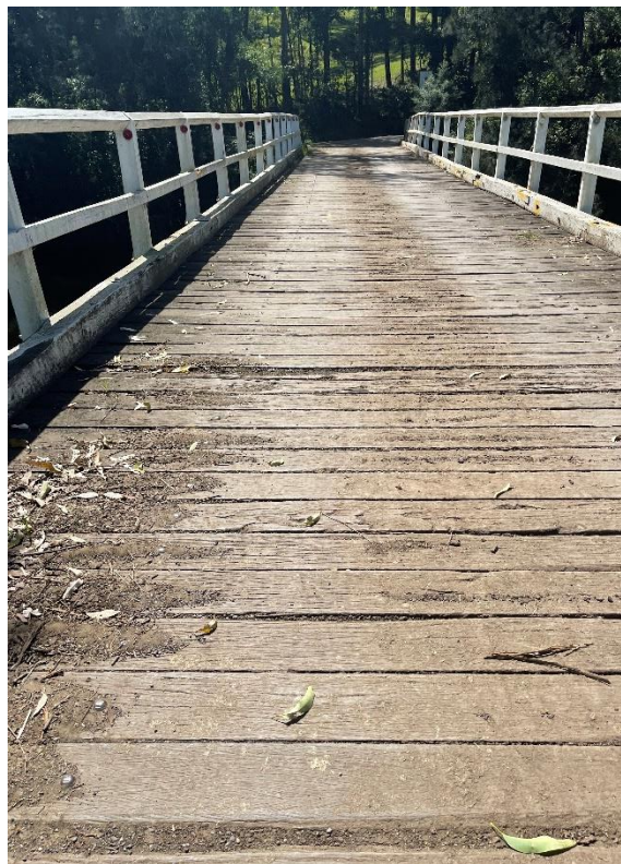
Figure 16. Decking and railings
